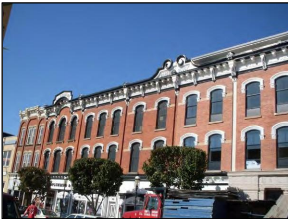
Barlow Block – 129 and 131-133 Main Street
