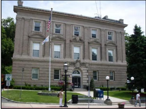
Ossining Municipal Building – 16 Croton Ave
