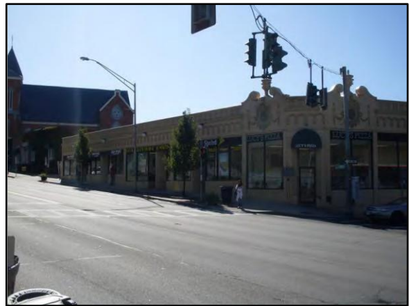
Cynthard Building - 30 South Highland Avenue
