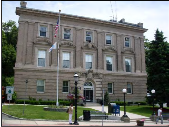
Ossining Municipal Building – 16 Croton Ave
