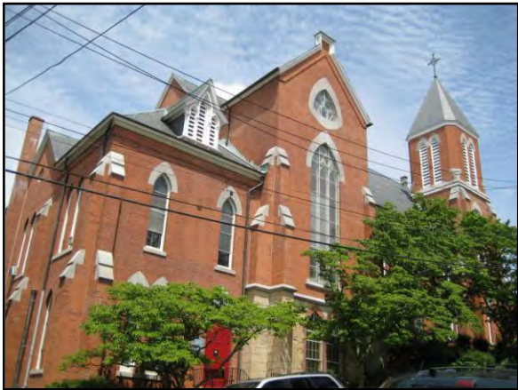
First Presbyterian Church – 34 S. Highland Avenue
