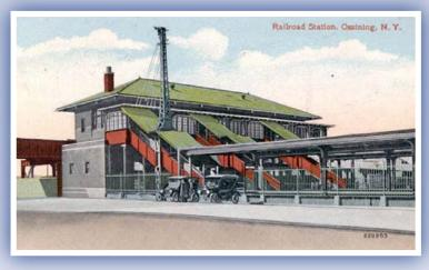
to the Village in 1851. Unlike the original station, which was located at-grade, the new Renaissance Revival-style station was built on metal stilts to allow Main Street to pass over the tracks and eliminate the need for a grade crossing. The station is sited above the tracks, spanning east to west, and is similar to stations that were built in Yonkers, Ludlow, Glenwood, and Hastings in the same time period.
