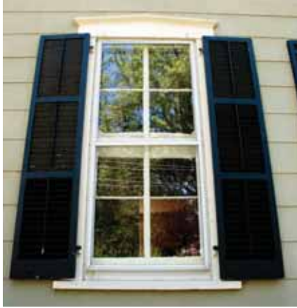
Above: correct installation of shutter and storm window; below: incorrect shutters.
