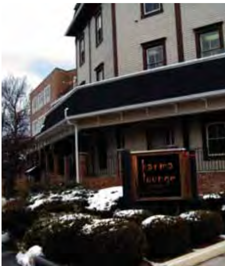
LEFT: Anachronistic and insensitive details such as brick piers, wrought iron railings, and white gutters compound the problems created by trying to fit a massive new element such as this covered walkway into an historic context.
