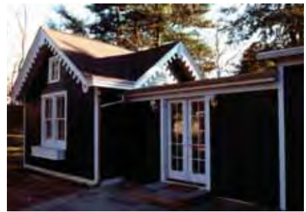
Connecting main structure and addition with a “hyphen” (see above and below) can help maintain an appropriate scale.
