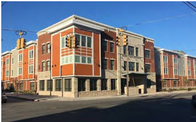
Cornice articulation on low-slope roofs
