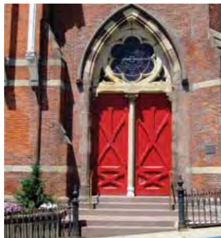
Successful historic entries consist of an assembly of elements including railing, step, molded surround and finally the doors themselves.
