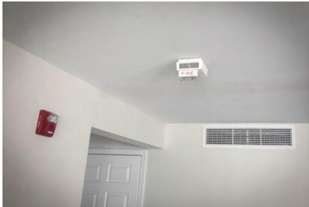
Fire alarm/smoke and CO detector strobe
