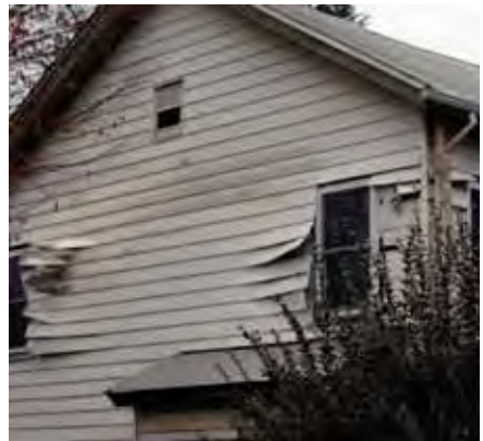
Visible history: it's worth looking for original clapboards still lurking under the more recent aluminum and asbestos layers.
