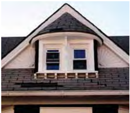
Original sunburst & special dormer details still carry the day in spite of roofing gaps and the reduced glass openings of replacement windows.
