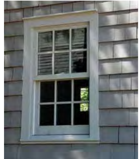
Above: a well-proportioned traditional double hung window, with head flashing, casing and sill.
