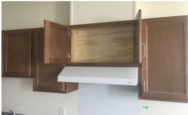
Boxed-in duct through range hood cabinet
