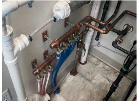
PEX System Manifold
