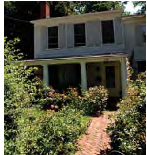
Sparta: porch shades the house, saving energy for cooling. Porous paving reduces runoff & recharges the aquifer.
