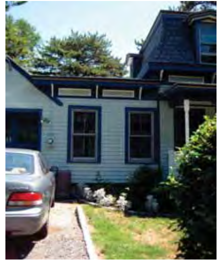
Connecting main structure and addition with a “hyphen” (see above and below) can help maintain an appropriate scale.
