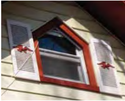
Above: correct installation of shutter and storm window; below: incorrect shutters.
