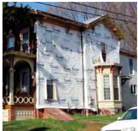
When re-siding try to create an air space under the siding with a smart air barrier to prolong siding life.
